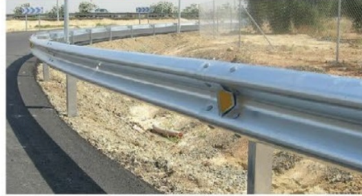
"W" BEAM CRASH BARRIER
