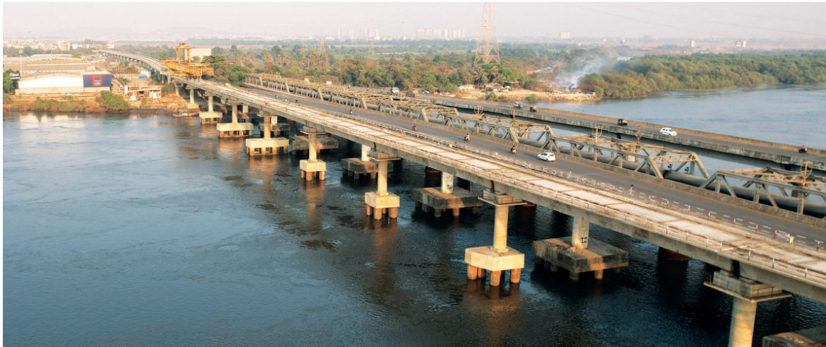
The Kasheli Creek bridge comprises 13 spans, including nine on water, with each span being 42.23 m in length with 15 segments.
