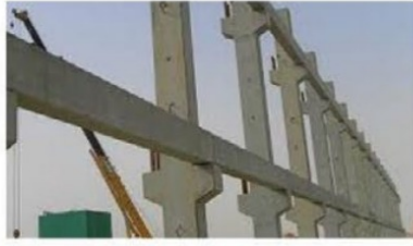
COLUMNS AND BEAMS
